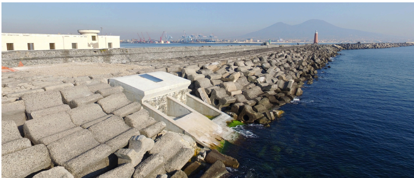
Prototype “OBREC” wave energy conversion system at the MaRELab (Marine Renewable Energy Laboratory)
