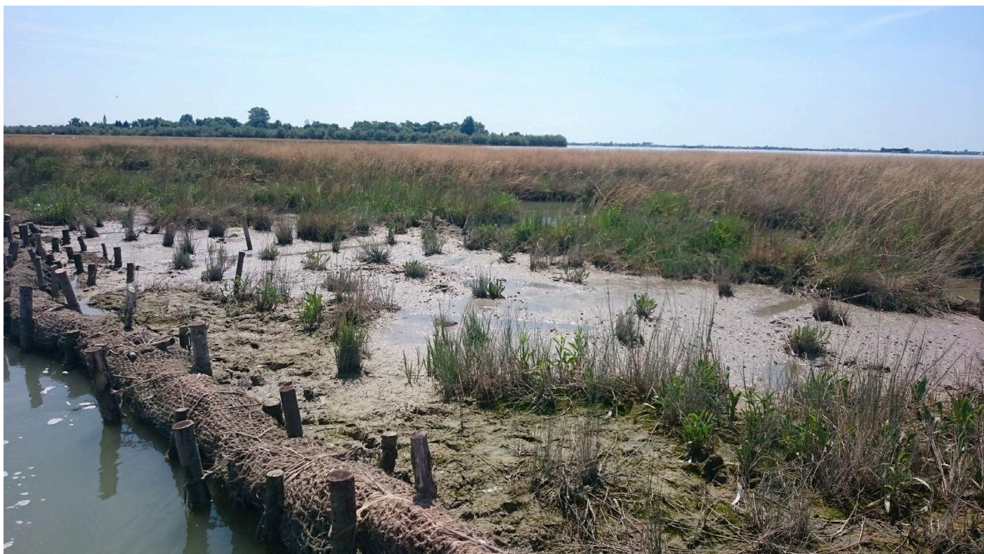
Nature based solutions against salt marsh erosion in the Lagoon of Venice (Italy), based on a combination of biodegradable barriers against waves and sediment nourishment to promote plant colonization. Credit: project LIFE VIMINE.
